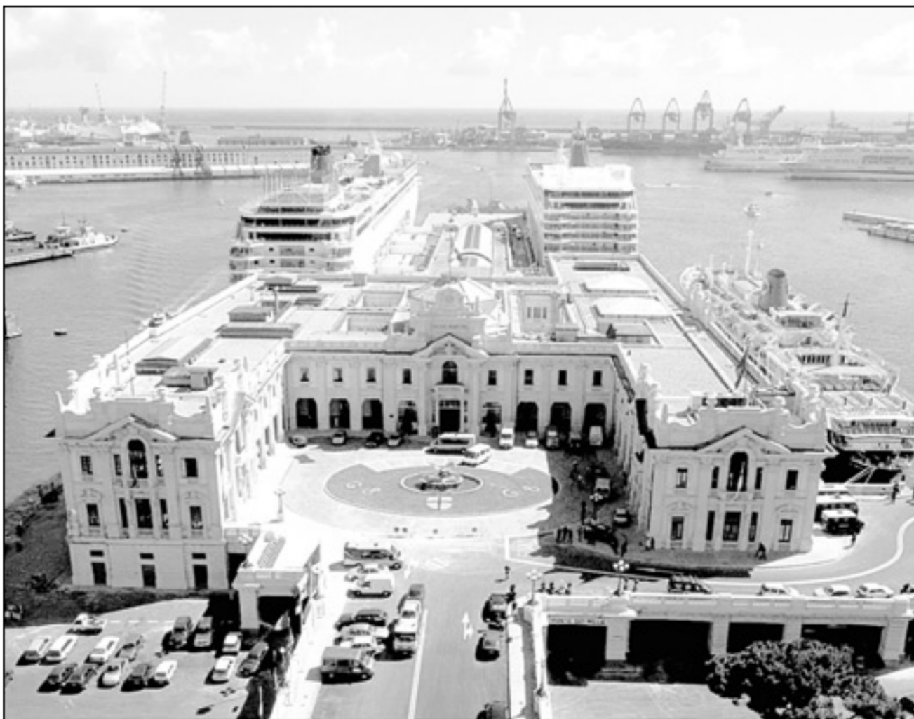
Ponte dei Mille Cruise Terminal in Genoa: commercial shipping made it more than just a backwater fishing port.
